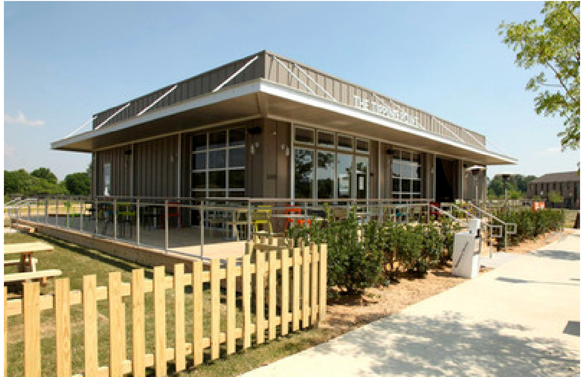
Moveable structure at Hampstead in Montgomery, Alabama. The structure can be unbolted into three pieces and relocated on flatbed trucks.
